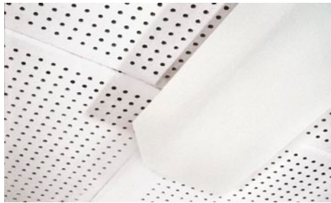
Perforated AIB ceiling tiles
