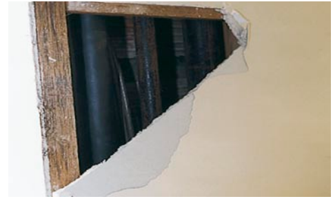
Asbestos insulating board (AIB)
